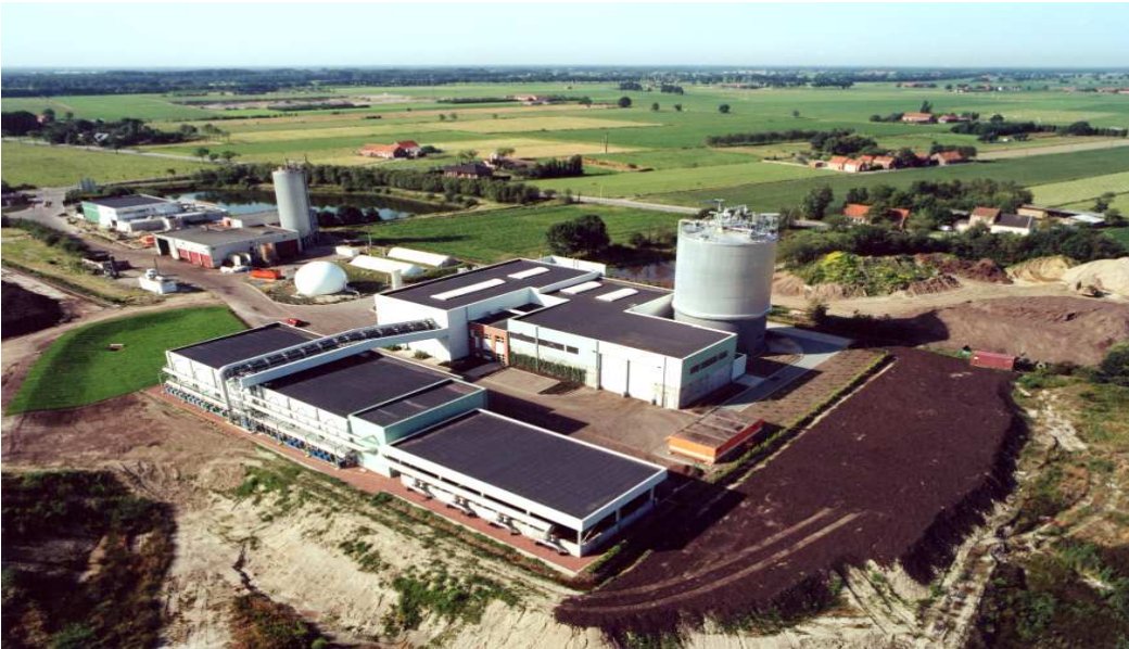
Figure 3: Dranco installation Brecht, Belgium
